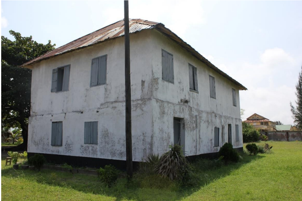
Figure S1. First storey constructed by Christian missionaries in 1845, Badagry, Nigeria (photograph by O. Adetunji).
