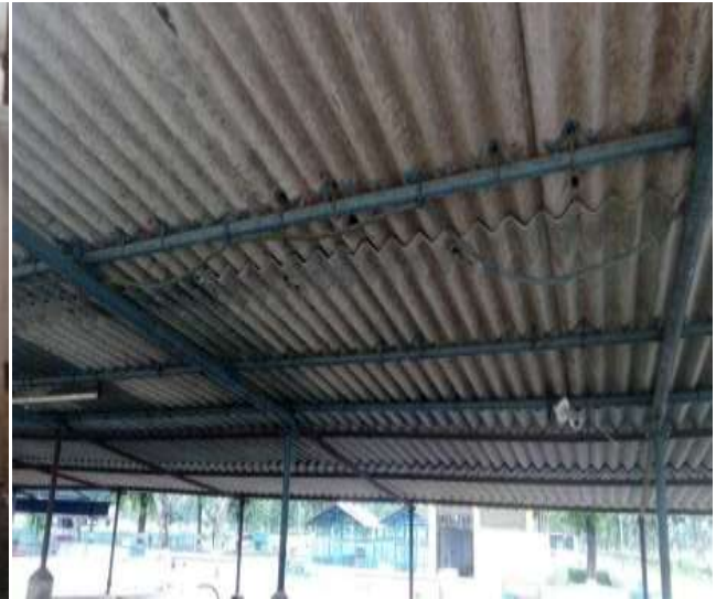
Asbestos roof
