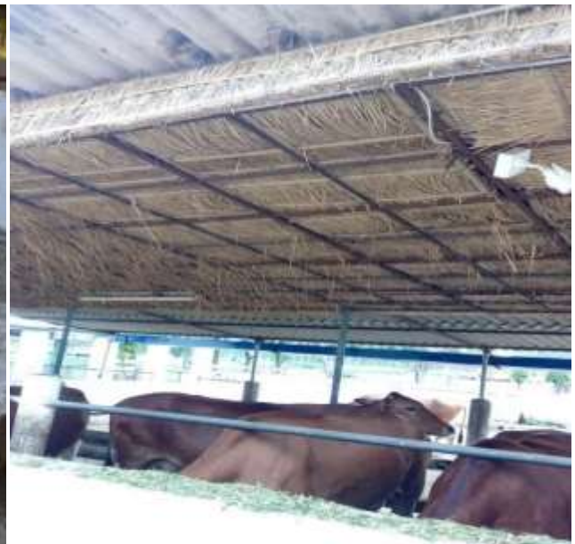
Thatched ceiling under asbestos roof
