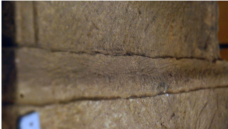
ONLINE FIG. 16. Poorly worked cyma recta on the front of the base. (Photo: P. Hill)
