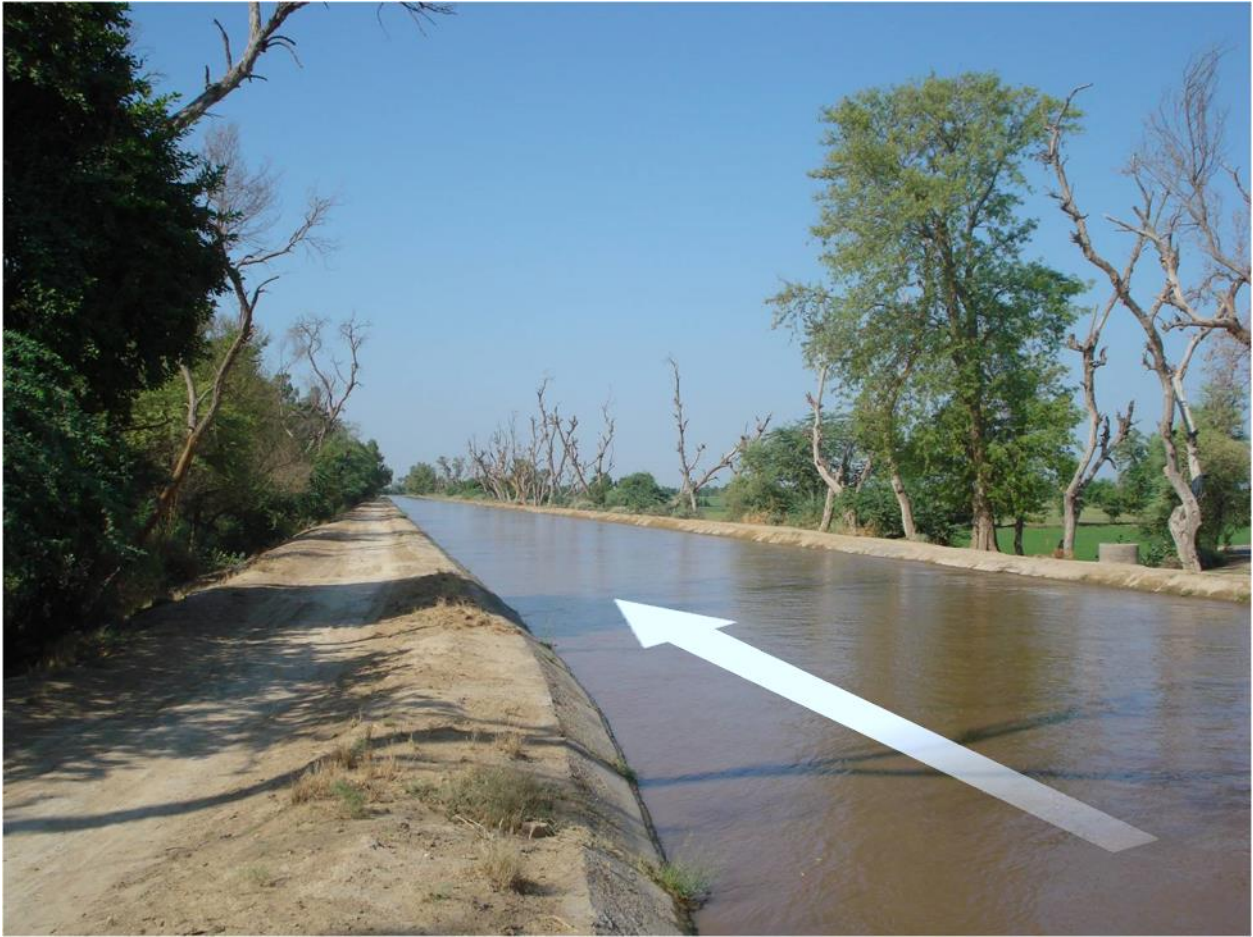
Figure A.2. A typical Hakra Branch Canal distributary channel (secondary canal) with direction of flow indicated
