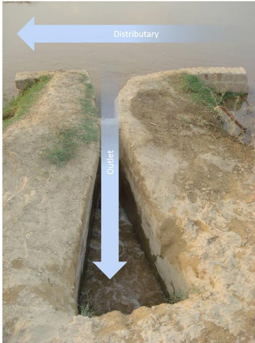
Figure A.3. A typical outlet structure on a Hakra Branch Canal distributary. Outlet draws water from the distributary channel. The size of the actual transmission structure (e.g. a pipe) is under ten inches with a designed discharge capacity under 10 cubic feet per second
